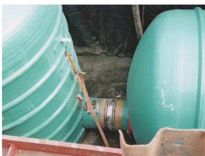
Flexseal coupling to connect all types of pipe up to 1200mm
