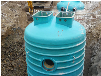
Large groutable inlet for concrete
